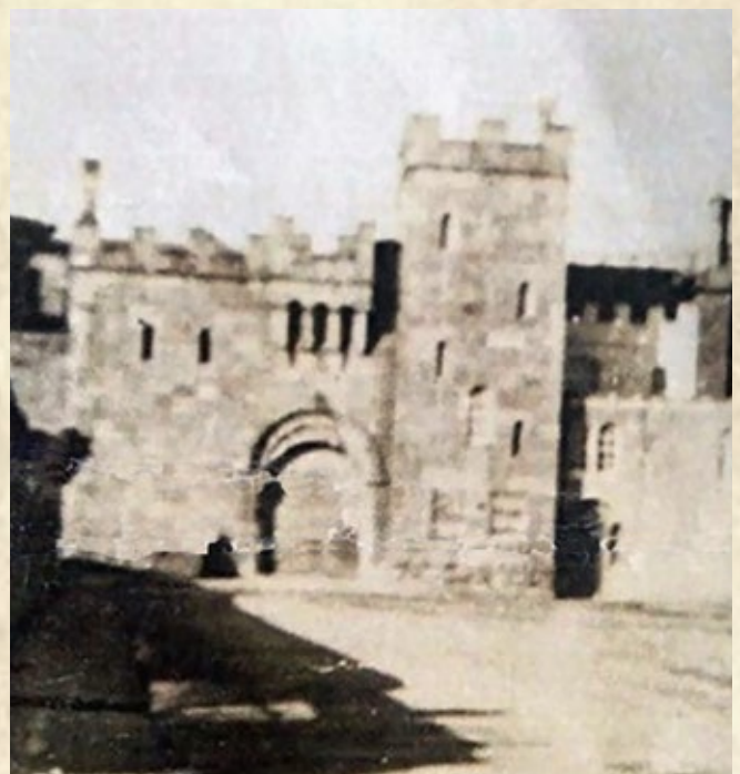
Kilkenny Jail, which was on St Riogh's Street, demolished in 1948
